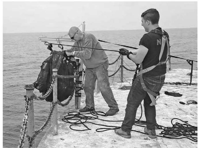
Matt Crehan and Jared Bergeron, N8CZ, hoisted the generator from the boat onto the lighthouse deck using the boom lift built by Jared and Nick Baine, AC8CQ.
